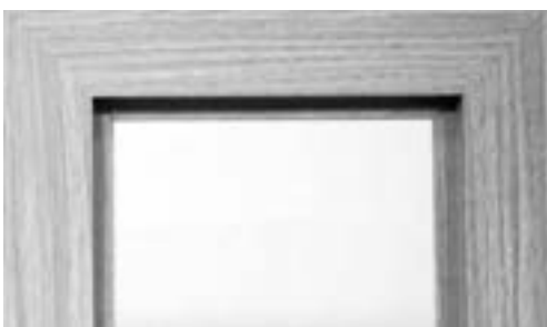
Back of door without glass installed, frame only
